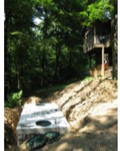
Our new septic system being installed courtesy of AWC Foundation Grant
