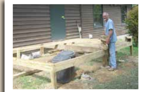
Ron builds our new deck
